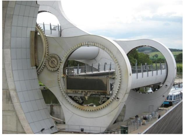
The rotation is controlled by a train of gears. It includes an alternating pattern of three 8 m (26 ft) diameter ring gears and two smaller idler gears, all with external teeth, as shown above. When the motors rotate the central axle, the arms swing and the small gears engage the central gear. The smaller gears then rotate at a higher speed than the wheel but in the same direction.
